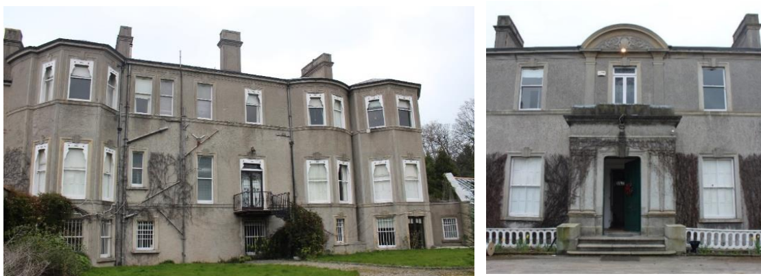
Fig.15.10: Rear Elevation (L), Entrance portico (R)
