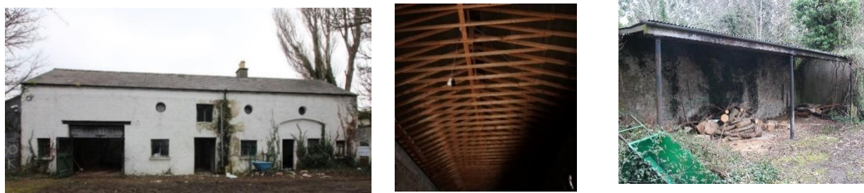
Fig.15.19: East elevation of stables (L), modern timber roof structure (M), Lean-to structure (R)
