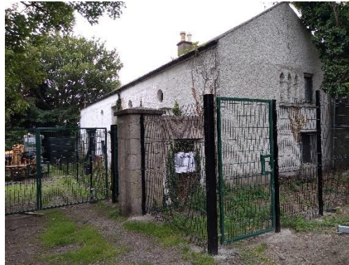
Plate 14.3 Coach house, facing southwest
