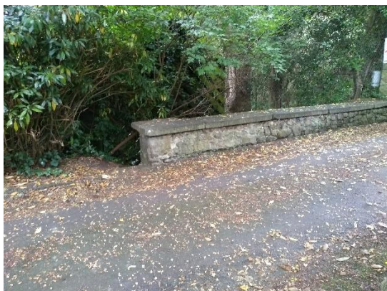
Plate 14.14 Bridge over townland boundary,
