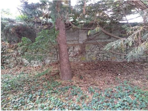
Plate 14.1 Southern wall, facing south
